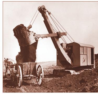
The Moore Speedcrane could be converted to operate as a crane, shovel, dragline or trench hoe. Here, one operates as a shovel in 1928..
